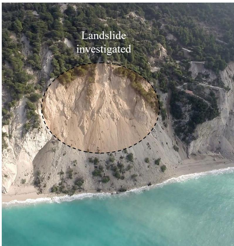
**Figure 1.** The major landslide triggered by the  $M_w$  6.5 earthquake at the site of Egremnoi (*Photo by [news.in.gr](http://news.in.gr)*)
