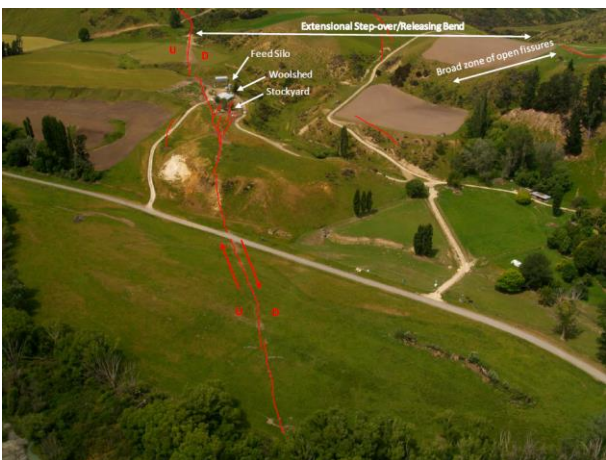
Figure 4: Aerial view of The Humps Fault surface rupture (red lines) at Glenbourne Farm, showing the sense of movement (red arrows) and highlighting farm infrastructure damaged by the earthquake (Lat 42.615°S, Lon 173.105°E; view northeast; photo and annotation by Clark Fenton).
