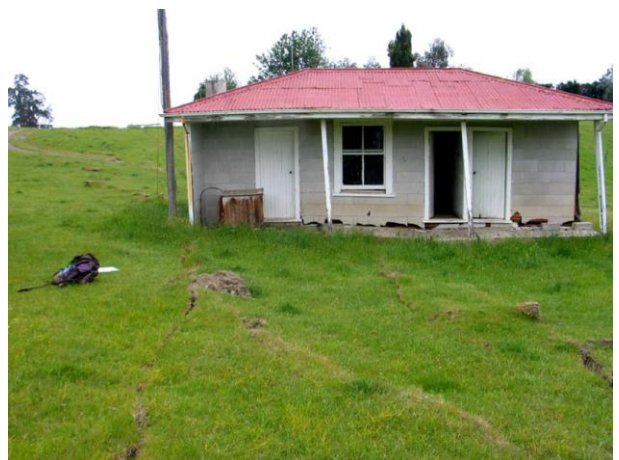
Figure 6: The Humps Fault surface rupture through a farm worker's cottage at Hossack Downs (Lat 42.629°S, Lon 173.015°E; photograph by Jarg Pettinga).
