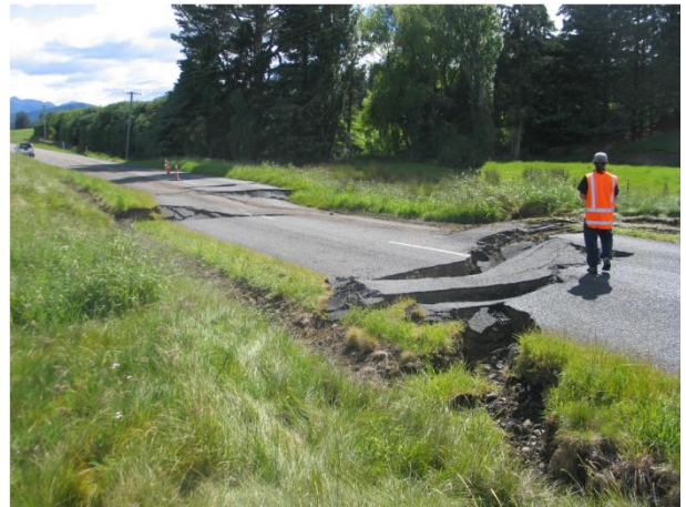
Figure 5: Oblique transtensional rupture within The Humps Fault zone displacing State Highway 70 (the Inland Kaikōura Road; Lat 42.597°S, Lon 173.091°E; view towards the north; photograph by Jarg Pettinga).
